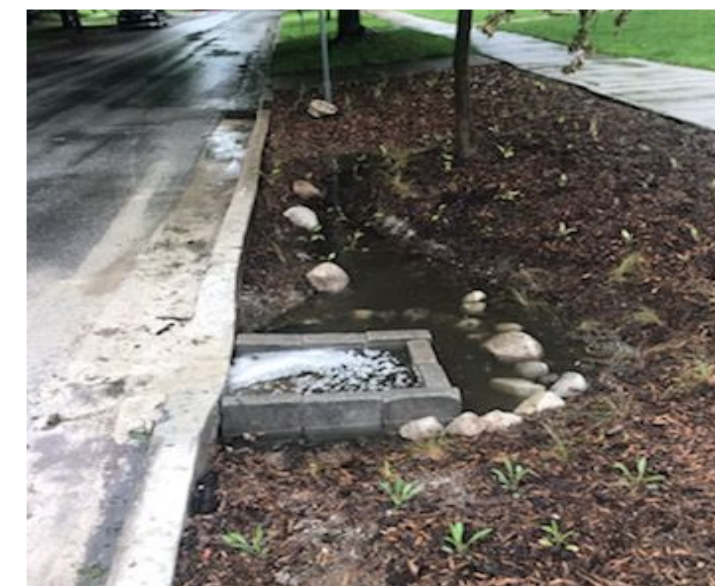
Fig. 3: A sediment trap in a rain garden filling with water, and depositing sediment into the trap that would have ultimately ended up in Plaster Creek.
