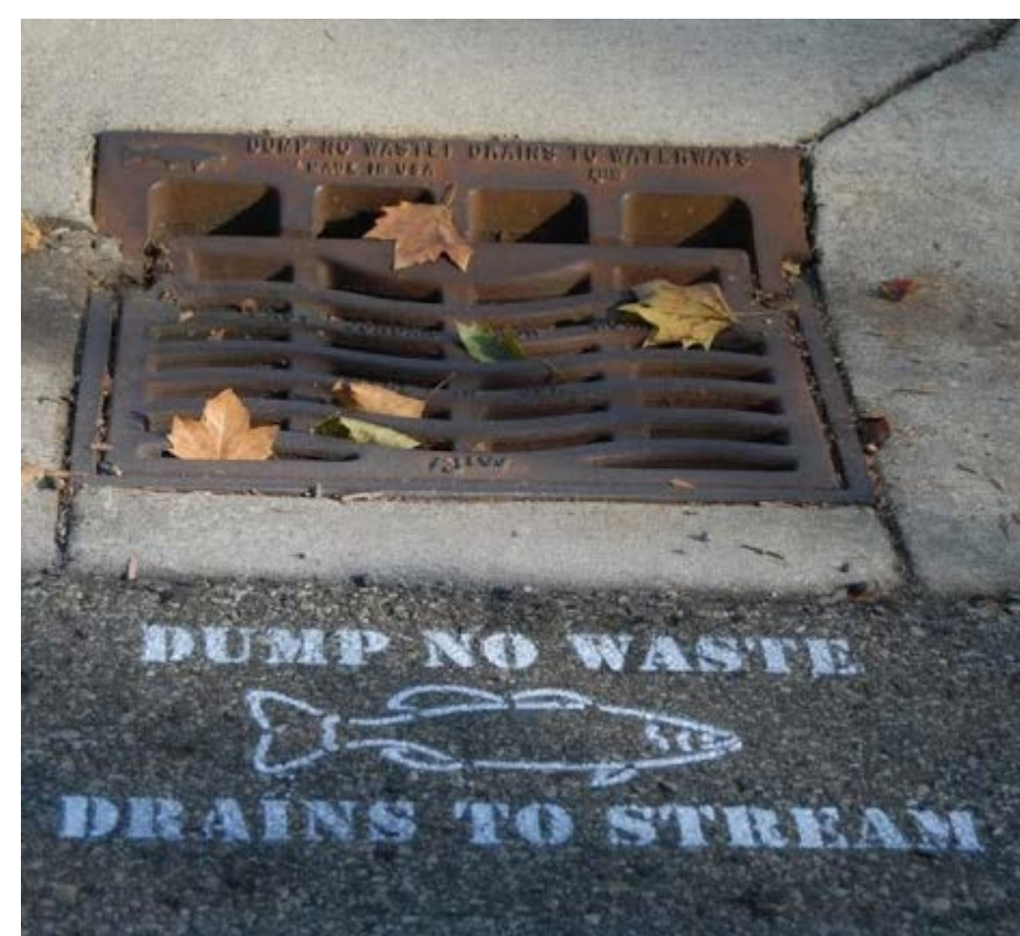
Stormwater catchbasin
