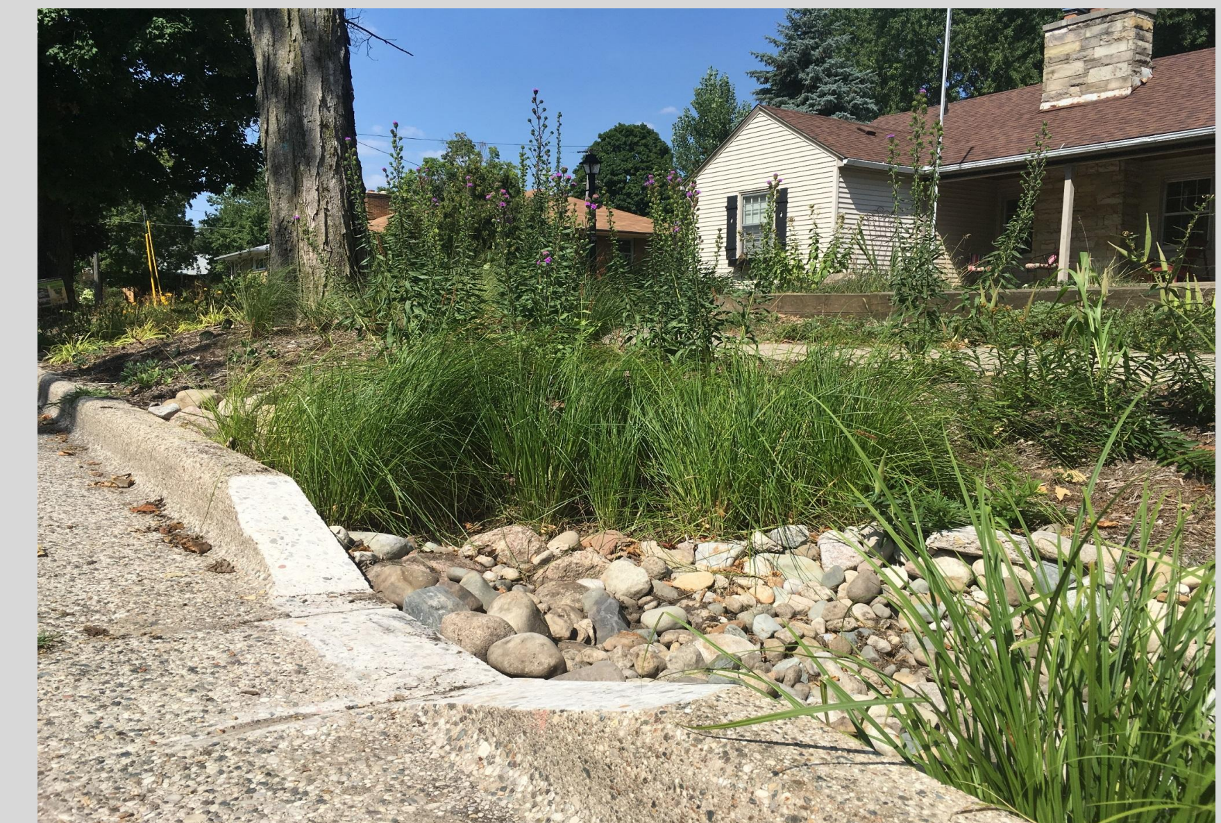
Figure 5: The cut curb of a mature rain garden in the Alger Heights neighborhood
