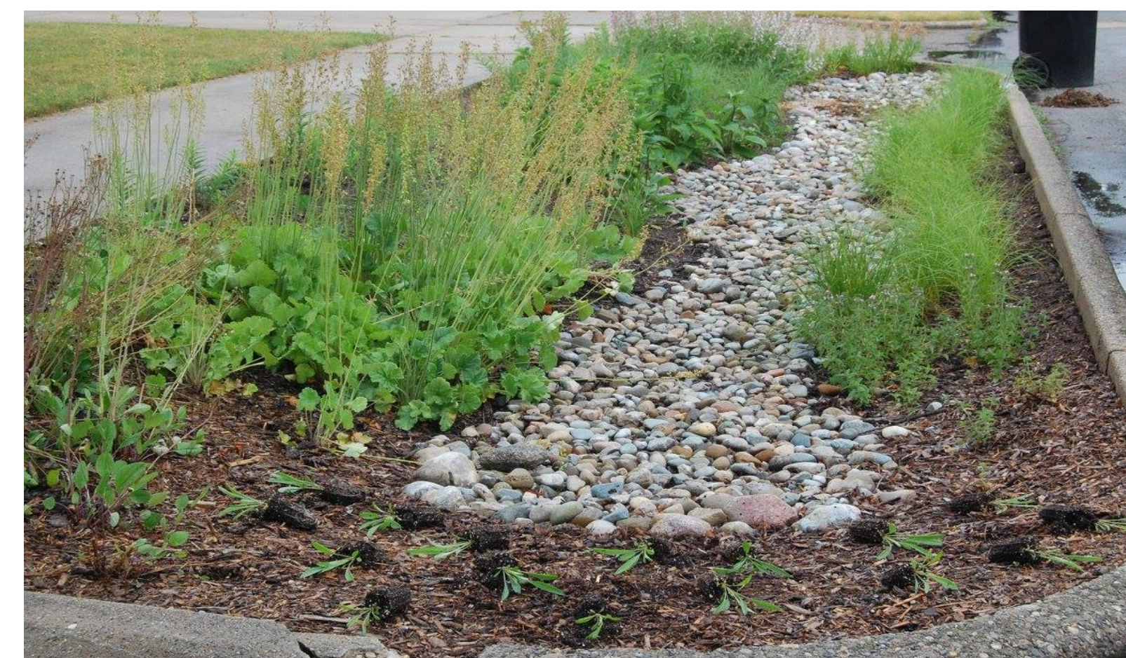
Fig. 1: A curb-cut rain garden installed by Plaster Creek Stewards. The rain garden consists of a rock channel with plantings around it
