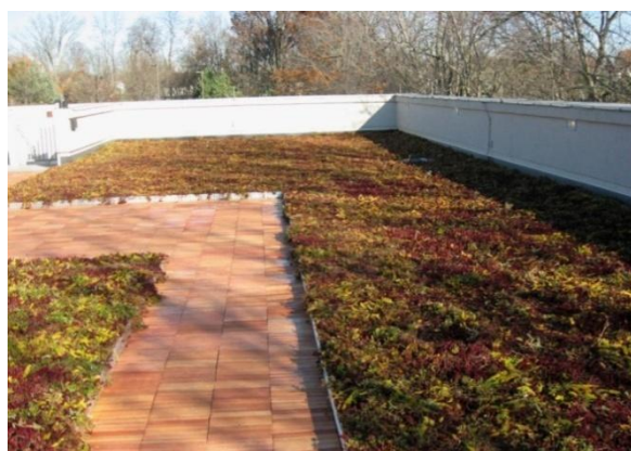
Figure 5-4. Green roof example.
