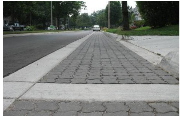
Figure 5-3. Porous pavement example.
