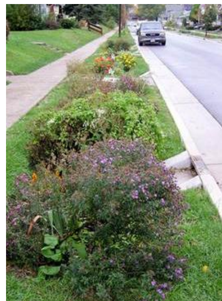
Figure 5-1. Linear bioretention example.
