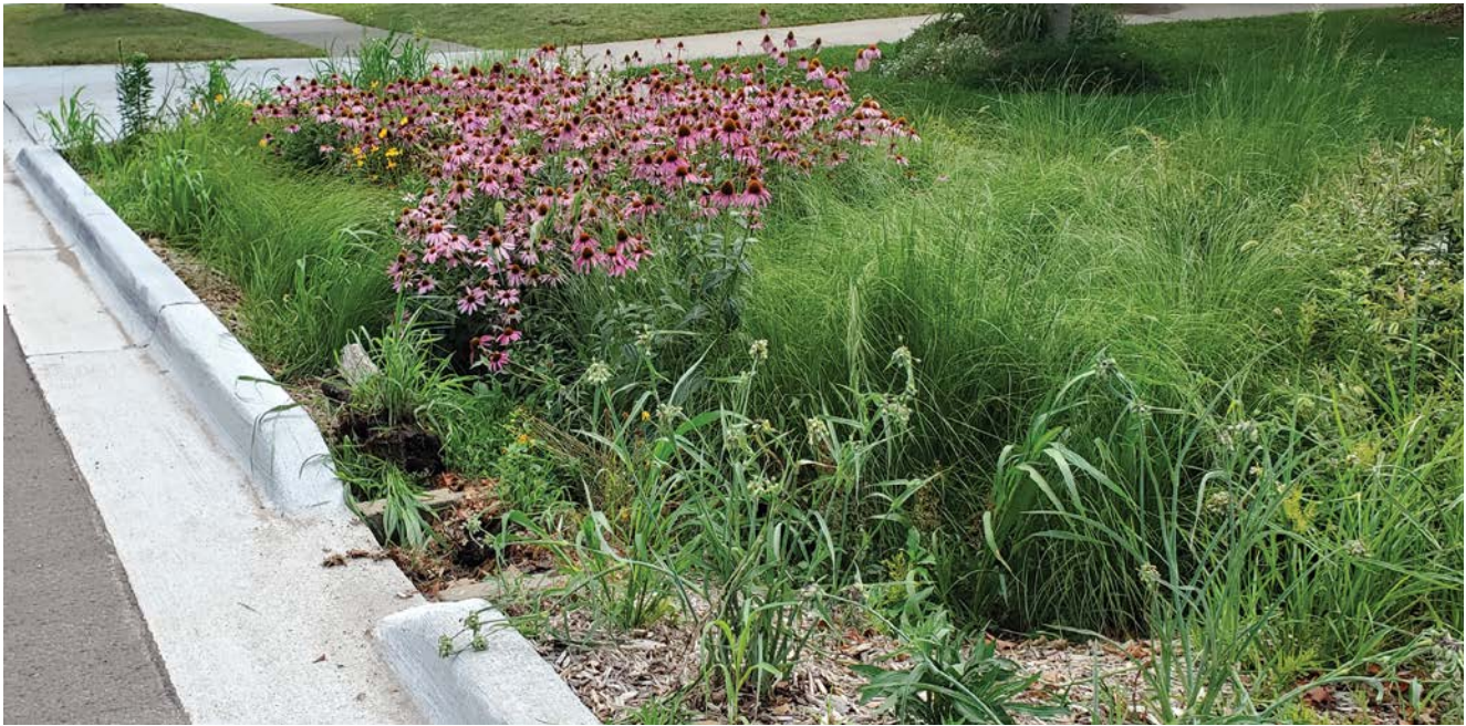
Figure 1. Example of a curb-cut rain garden one full growing season after initial planting. Water moving along the curb destined for a storm drain becomes diverted into the garden, where the curb has been cut. Debris and sediment are captured within the concrete pavers. The water continues to flow into the basin where it slows down, percolates into the soil, evaporates, or is transpired by native plants in the garden.
