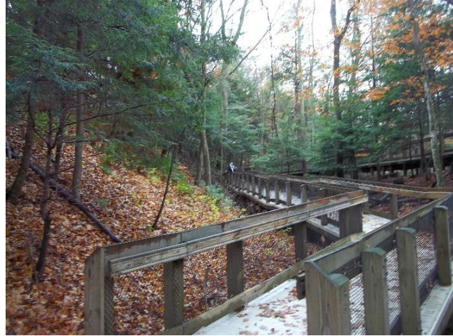
Figure 6. Metal section of the boardwalk.
