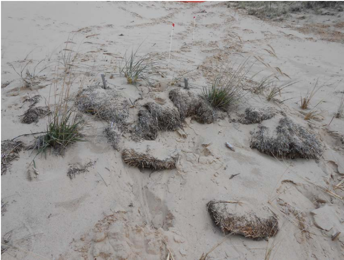
Figure 5: Straw bales placed on the dune in 2009 for surface stabilization remain present in 2012. Photo taken November 2012.
