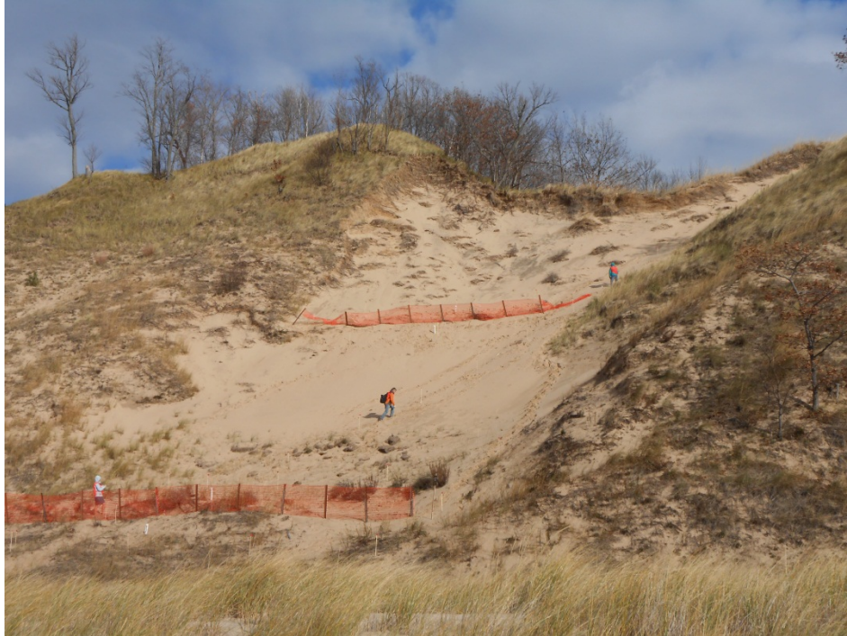
Figure 3: View of windward slope of Castle Park Dune showing the 50-meter high blowout and the two sand fences installed in April 2012. Photo taken November 2012.
