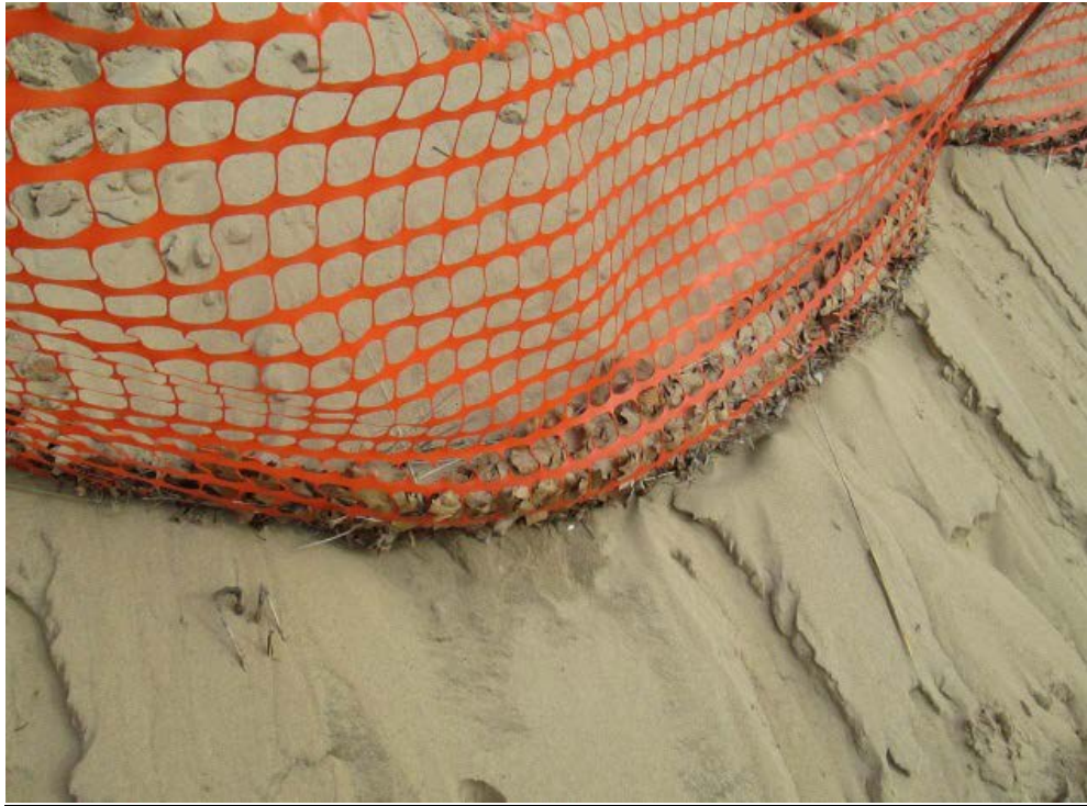
Figure 11: Deposited sand easily slid under the flexible plastic netting of the sand fences. Photo taken November 2012.
