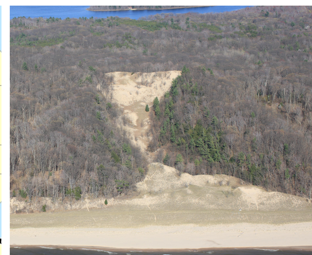
Figure 2: An oblique aerial view of Dune 2, U.S. Army Corps of Engineers 2012 .
