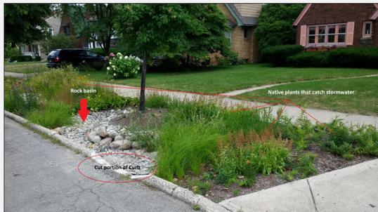
Figure 1: In a curb-cut rain garden stormwater runoff enters into a rocky basin through a literal cut in the curb; native plants assist in filtering and evapotranspiring the trapped rainwater.
