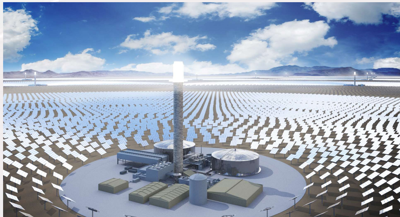
Model of a concentrated solar power tower system with a heliostat field. This is the type of CSP system we are analyzing.
